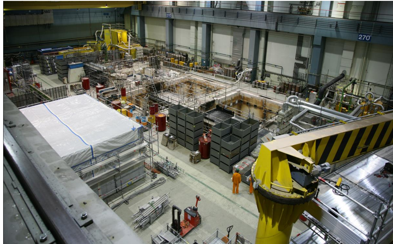
Waste Treatment Center in Turbine Hall of Würzgassen NPP (Boiling Water Reactor)
