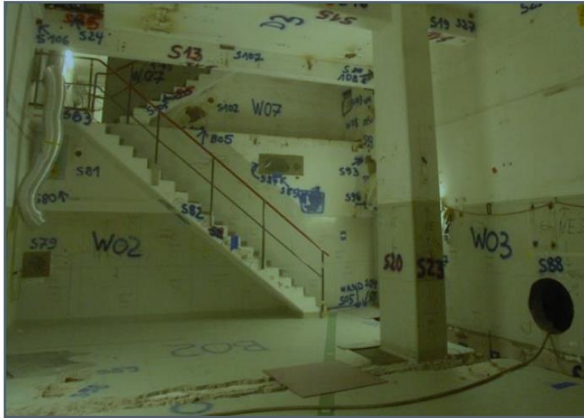
Figure 6: Room to be measured for clearance with sampling points (PreussenElektra GmbH, Würgassen nuclear power plant)
